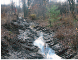
Mimicking sinuosity and preserving connection to flood plain in the dredged section of the stream.
