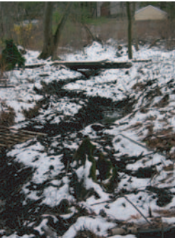
Hand dug portion of upstream channel mimicks natural downstream morphology.
