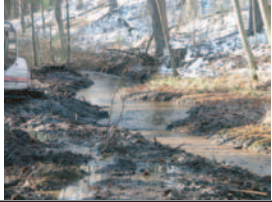
Create a channel with a connection to its flood plain. Incorporate meanders to promote dissipation of energy.
